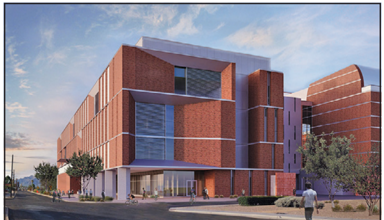
The Bioscience Research Laboratory Building will provide much needed space for interdisciplinary research.
