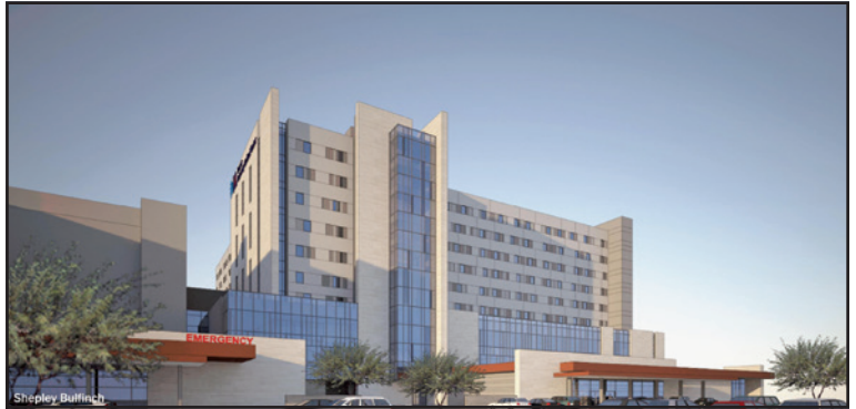
The new 670,000 sq. ft. University Medical Center Tucson is expected to be completed in 2019.
